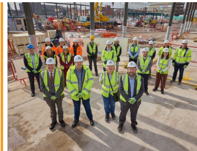
VIP guests with Councillor Anthony Burns, Leader of St Helens Borough Council in March 2026, help secure the final bolt on the new bus station steel framework
