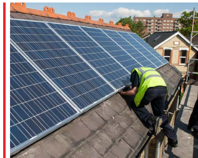
Engineer installing solar panels on a roof
