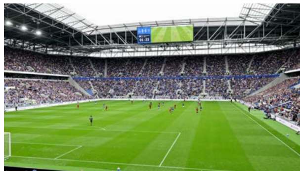
Inside Hill Dickinson Stadium
