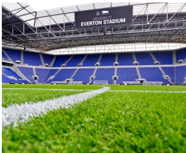
A view from the turf at Hill Dickinson Stadium
