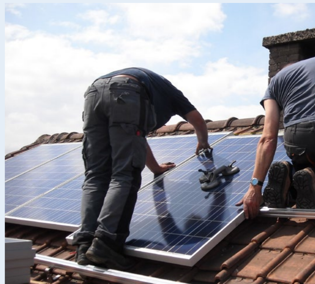
Installation of solar panels
