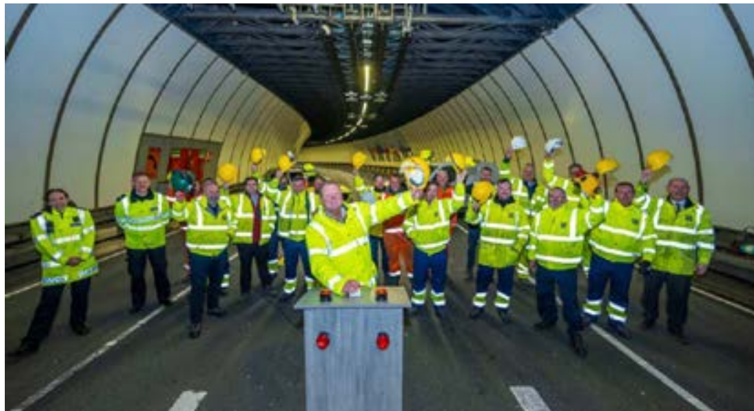
Clr Steve Foulkes officially switches on the new LED lighting system alongside members of the project team who made it happen.
