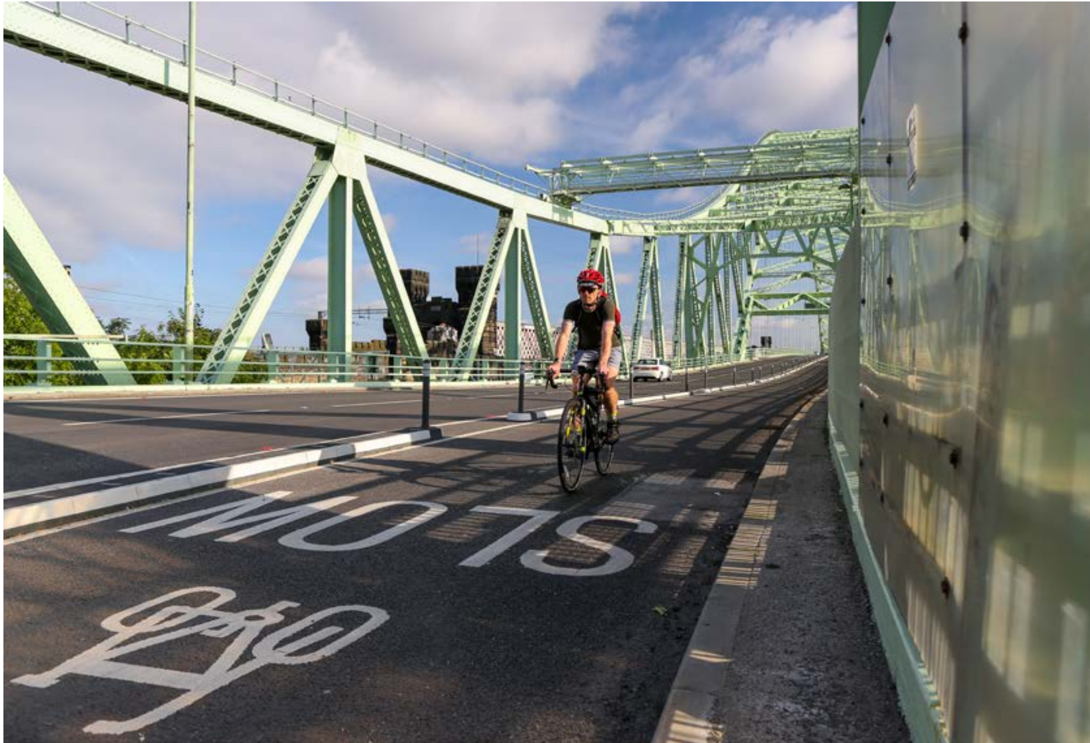
The segregated cycleway on the Silver Jubilee Bridge in Widnes.
