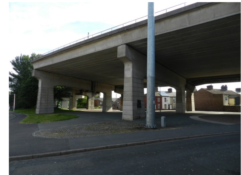
Runcorn Approach Viaduct
