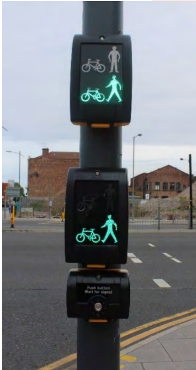
Figure 3.5: Toucan crossing, Leeds Street, Liverpool
